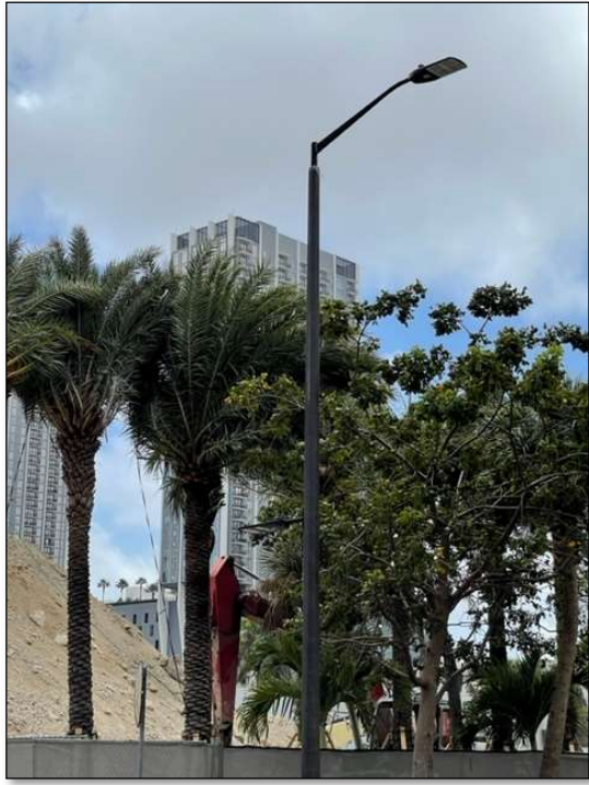
EXISTING UTILITY – LIGHT POLE
