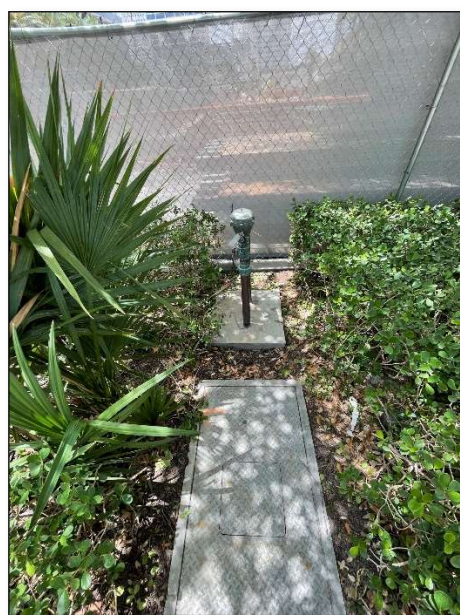
EXISTING UTILITY – 2" IRRIGATION METER
