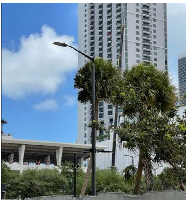
EXISTING UTILITY – LIGHT POLE
