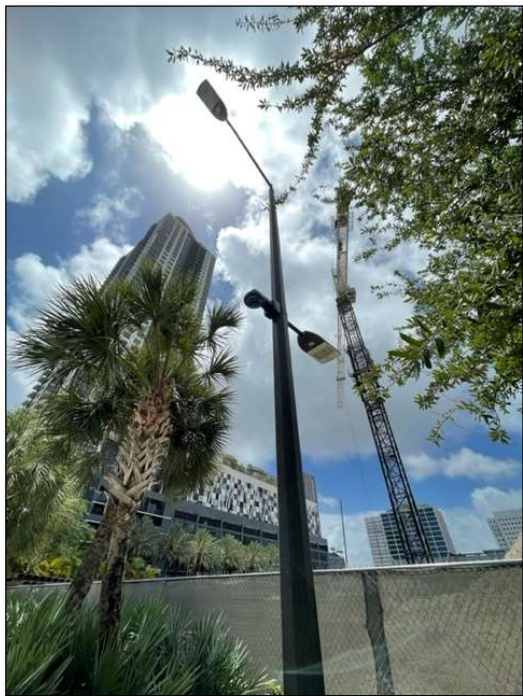
EXISTING UTILITY – LIGHT POLE WITH CAMERA
